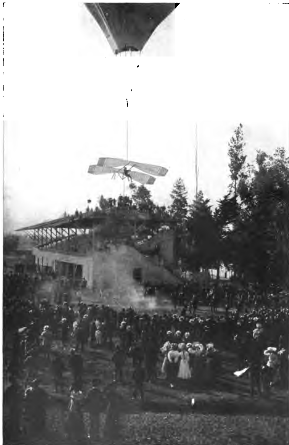
FIGURE 173.—Elevating Montgomery Aeroplane with a balloon, in California, in 1905.
