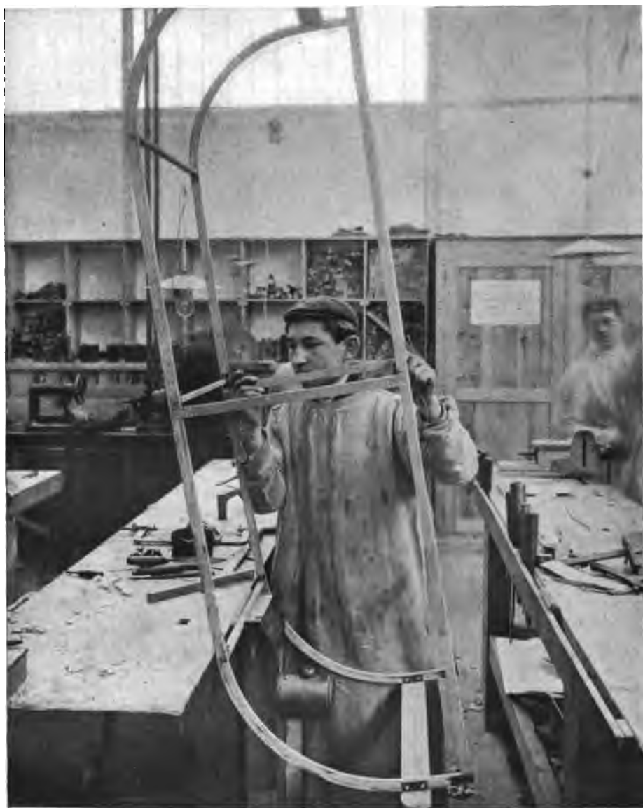
FIGURE 195.—Rudder Frame of Wright Machine.
