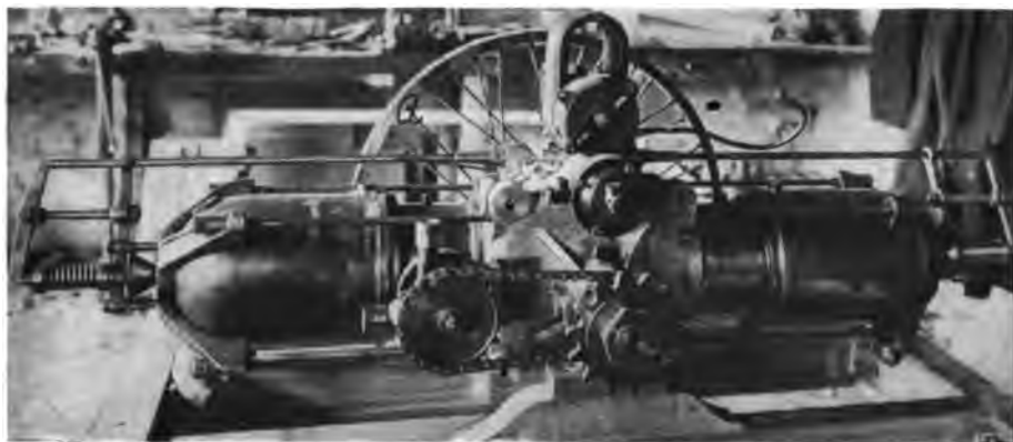
FIGURE 115.—Flat and Panhard Aeronautical Motors. These are remarkable examples of refined construction, the Flat developing 50 horsepower with a weight of only 110 pounds, and the Panhard weighing 176 pounds for 45 horsepower.
