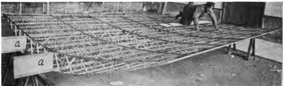
FIGURE 72.—Framing of Antoinette Wing Inverted. The load is supported on the two main girders aa , which are connected by a maze of crossbraces to the transverse ribs and secondary longitudinal members.
