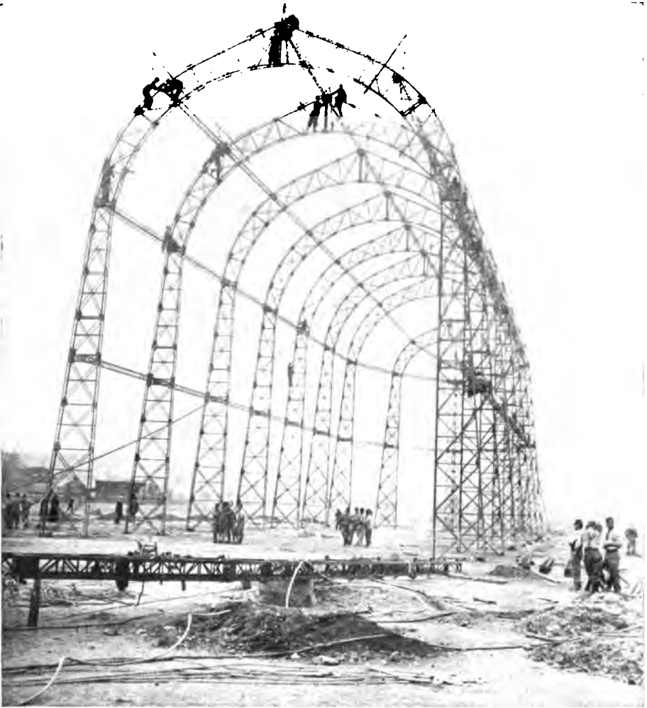
FIGURE 15. —Portable Balloon House Used by the French Army. This immense structure is built in easily assembled and dismantled units, so that it can be hauled to a desired point by wagon train and quickly set up. Note the arch on the ground, awaiting erection.
