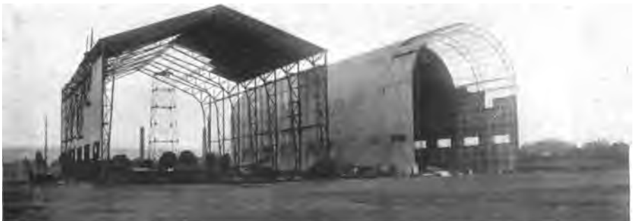
FIGURE 16. —Balloon Houses Nearing Completion.
